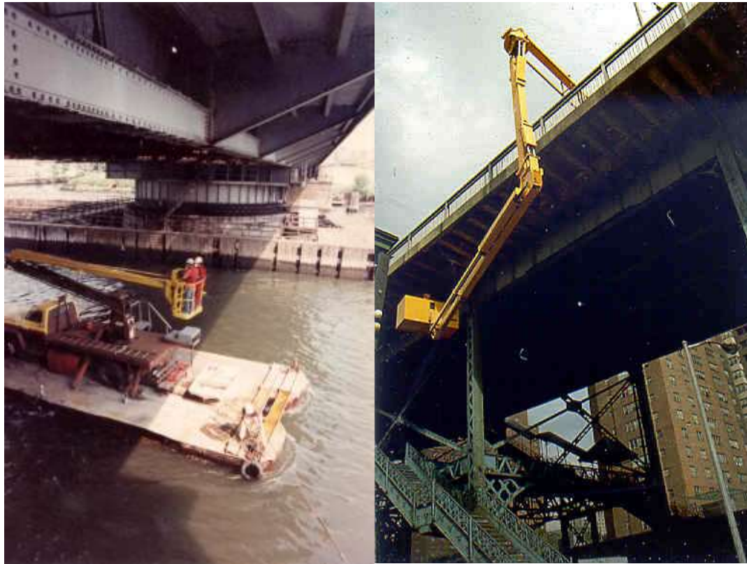
Manual inspection using a movable inspection gondola
